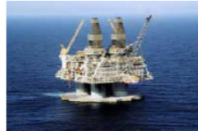
<Exploration and Production of the Natural Gas>
