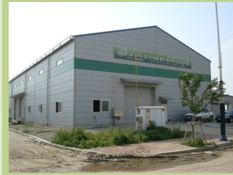
Construction of building (2010)
