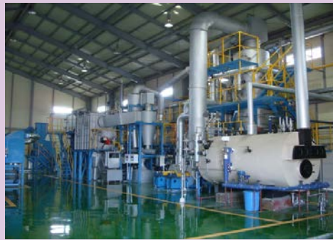
Manufacture of gasification facility(2011. 05)
