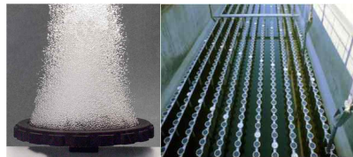
< Fine pore diffuser >
