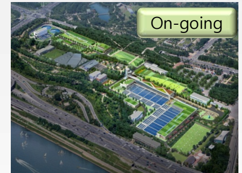
Dookdo Purification Facility
