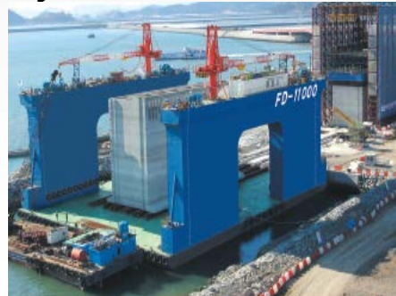
Ulsan New Port (Caisson)
