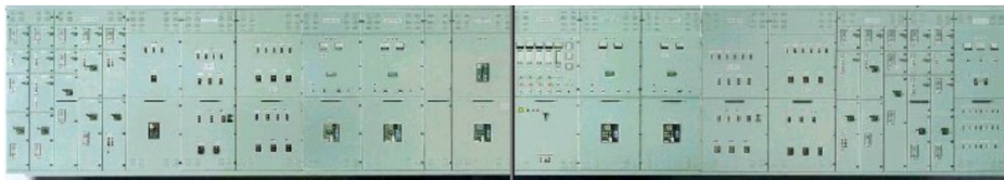
Example of switchboard
