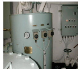
Hot Water Calorifier
