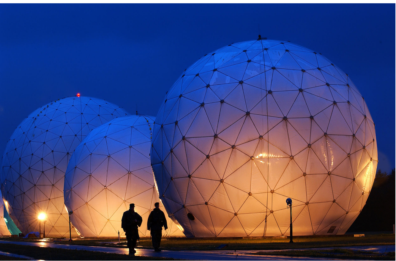
Radome (Radar + dome) permits EM waves through enclosure with little reflection
