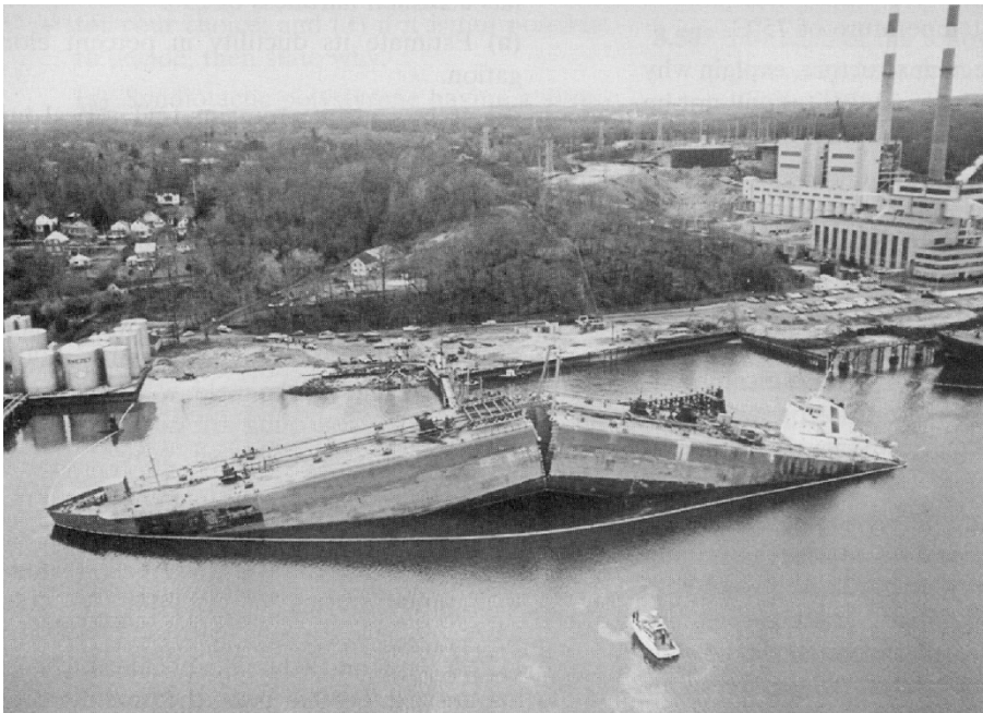
Oil tanker fractured in a brittle manner
