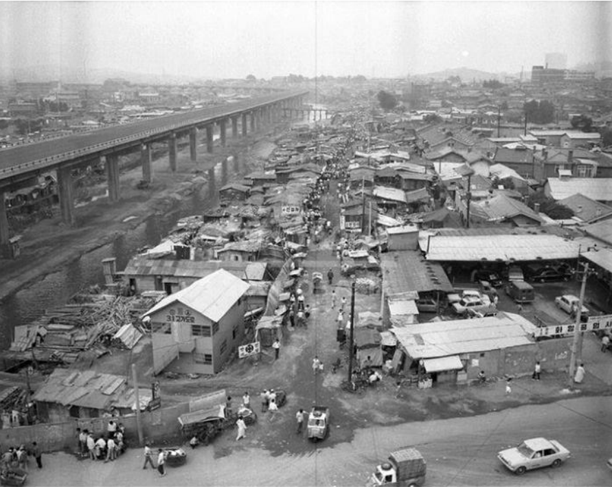
Cheongyecheon before covering
