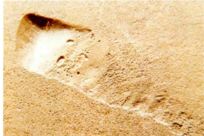
Figure. Erosion Site on Pipeline Wall
