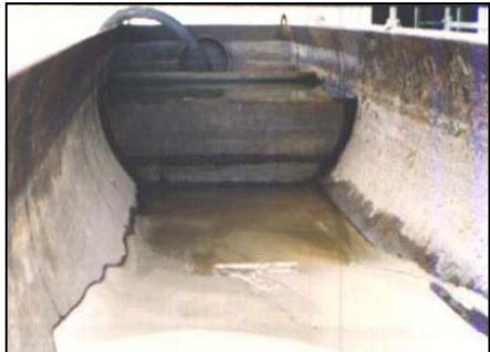
Sand Plugging (especially at CV)
