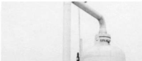
Figure 1-1. A typical vertical two-phase separator at a land location. The inlet comes in the left side, gas comes off the top, and liquid leaves the bottom right side of the separator.
