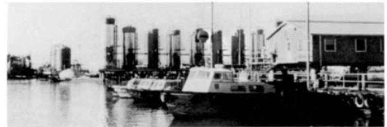
Figure 1-32. A marsh facility where the equipment is elevated on concrete platforms. Note the two large vertical separators in the distance, the row of nine vertical heater treaters, and the elevated quarters building.
