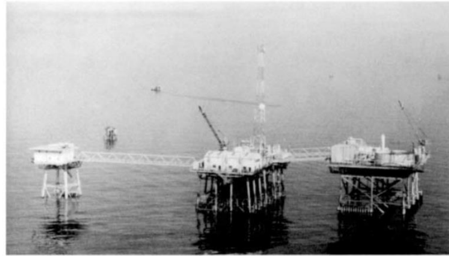
Figure 1-36. In moderate water depths it is possible to separate the quarters (on the left) and oil storage (on the right) from the rest of the equipment for safety reasons.
