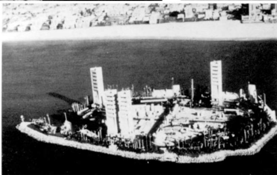
Figure 1-41. Sometimes the facilities must be decorated to meet some group's idea of what is aesthetically pleasing. This facility off California has palm trees, fake waterfalls and drilling derricks disguised as condominiums.
