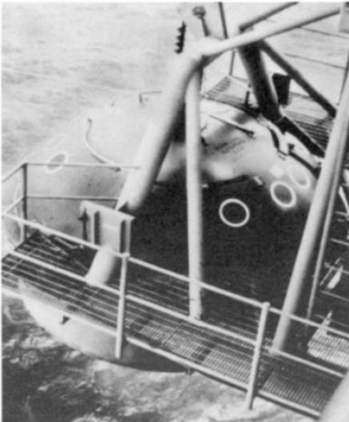
Figure 1-24. An escape capsule mounted on the lower deck of a platform. The unit contains an automatic lowering device and motor for leaving the vicinity of the platform.
