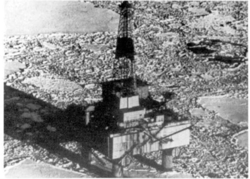
Figure 1-38. In cold weather areas such as this platform in Cook Inlet, Alaska, the facilities may be totally enclosed.
