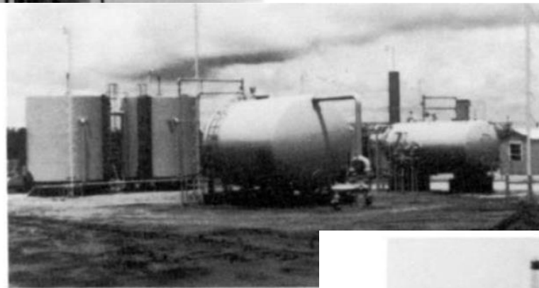
Figure 1-31. An onshore central facility with a knockout, and a horizontal heater treater.
