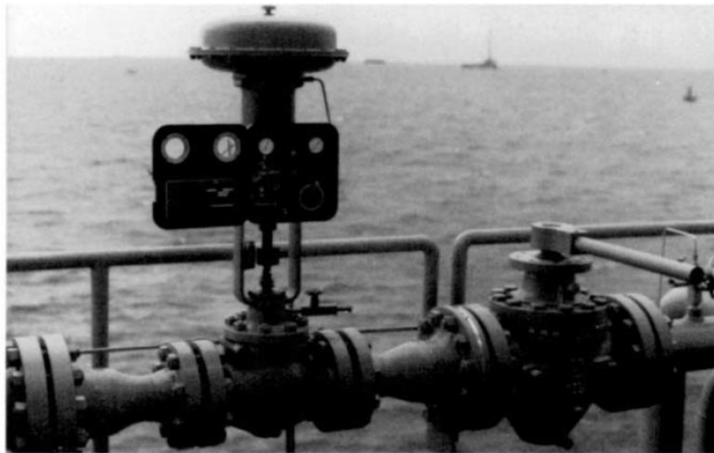
Figure 1-25. A pressure control valve with pneumatic actuator and pressure controller mounted on the actuator. The control mechanism in the box senses pressure and adjusts the supply pressure to the actuator diaphragm causing the valve stem to move up and down as required.
