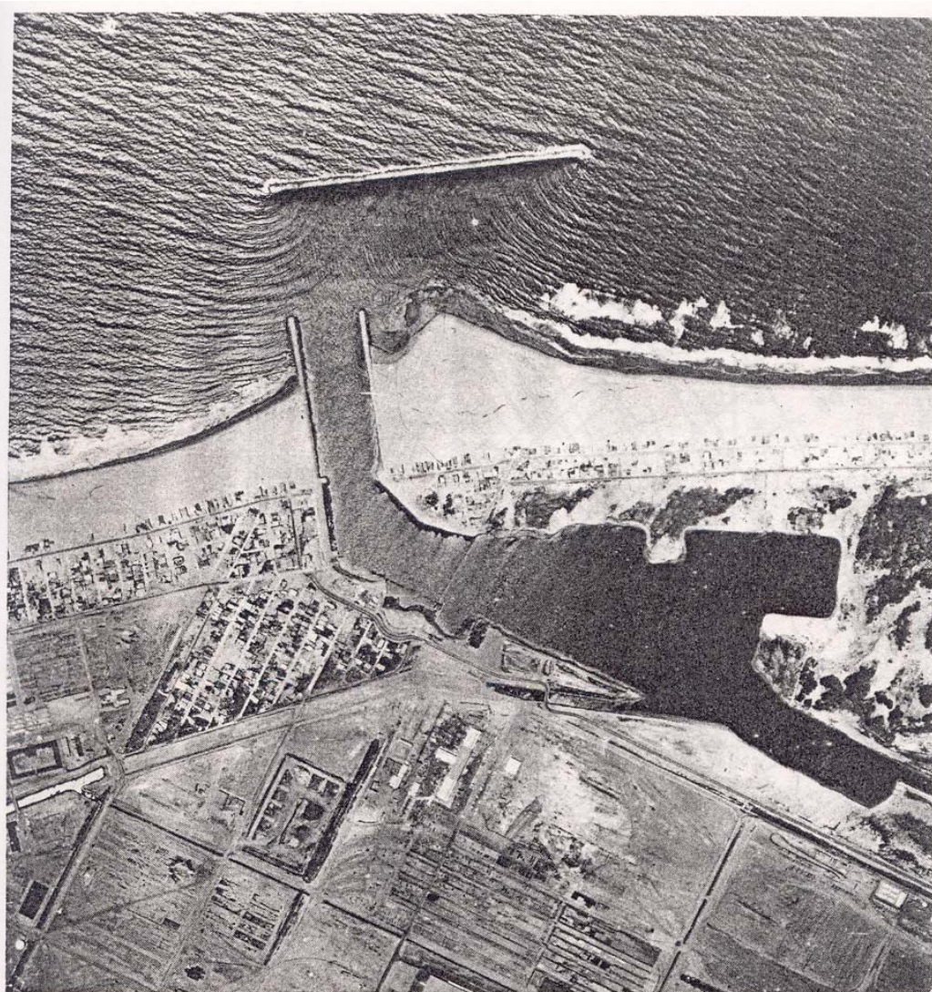
Figure 2-27. Wave diffraction at Channel Islands Harbor breakwater, California.
