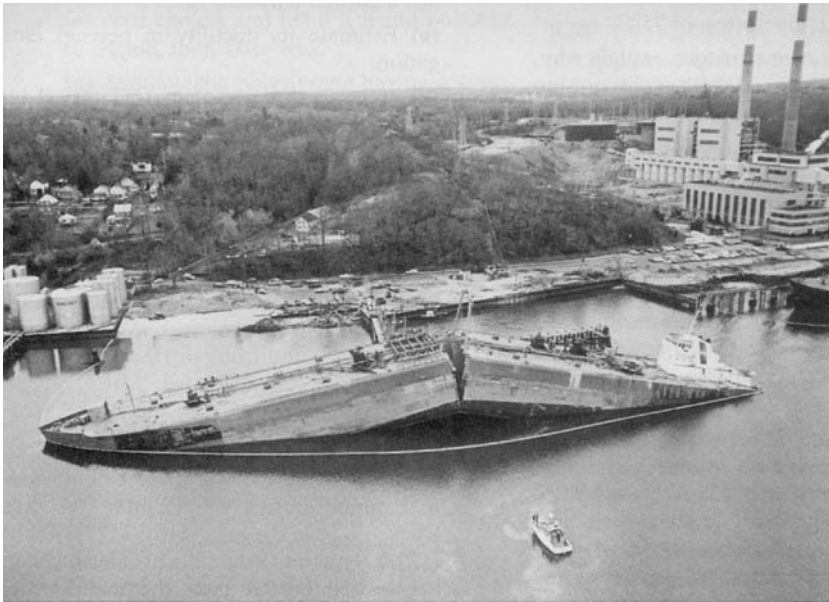
Oil tanker fractured in a brittle manner
