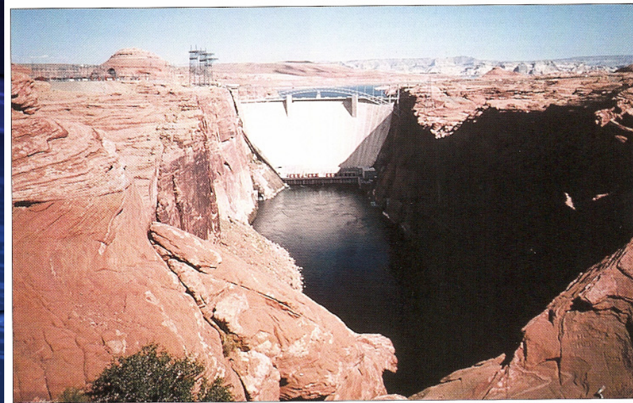
● FIGURE 14.26 Glen Canyon Dam hydroelectric project. In dry surroundings such as these, evaporation losses from reservoirs are high and can exacerbate regional water-supply problems.
