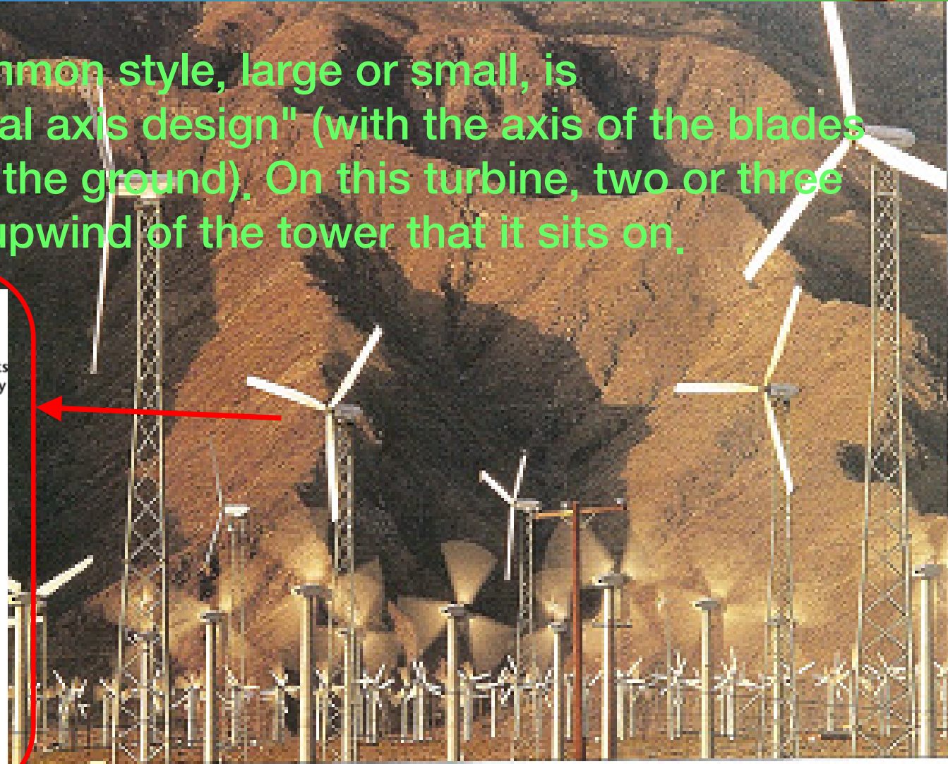
FIGURE 14.31 Wind-turbine array near Palm Springs, California. Different elements of the array can take advantage of various velocities of wind. Some of the smaller turbines are turning even in light wind, while the larger turbines require stronger winds to drive them. © The McGraw-Hill Companies, Inc./Doug Starnes, photographer.
