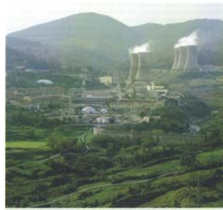
Figure 9.3 The Larderello 3 station, which produces 120 MW from six turbine units. The geothermal pipeline network consists of an inner steel pipe lagged with asbestos fibre and covered with aluminium plates.
