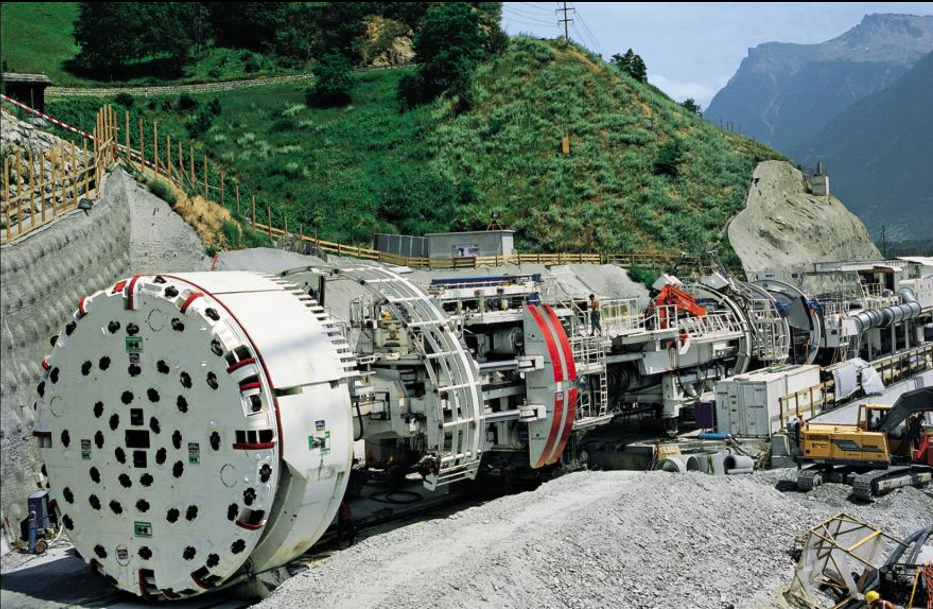
Hard Rock TBM
