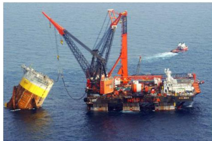
Upending of Spar Hull by Heerema HLV (Balder)
