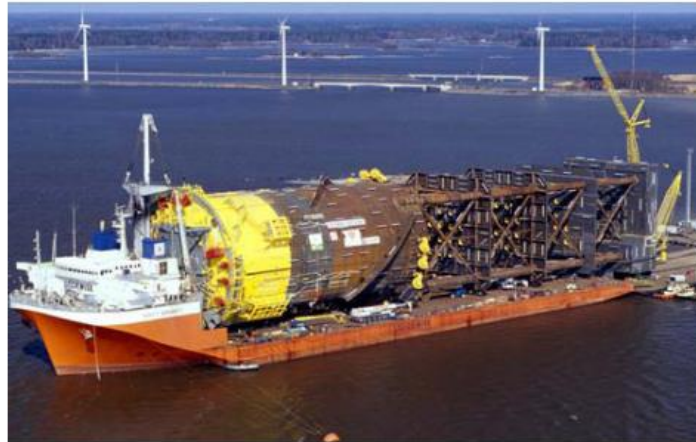
Dry-transport of Spar Hull
