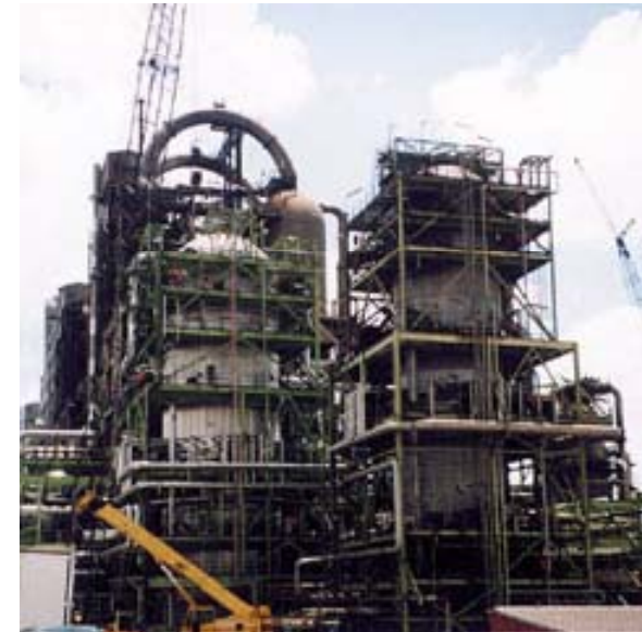
GTL reactor for Sasol coal-gasified gas into synthetic oil
