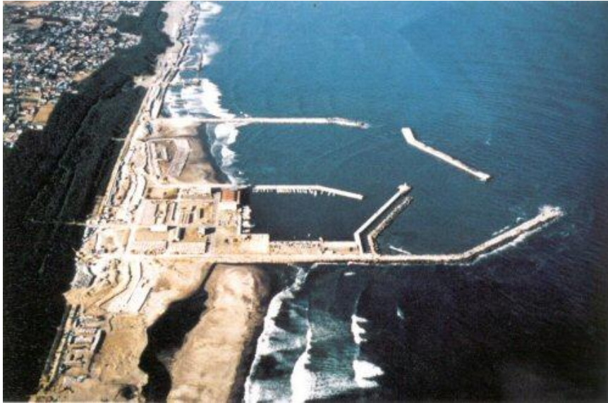
Breakwater for harbors
