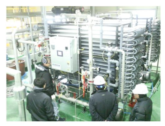
Tubular UF membrane for solid separation
