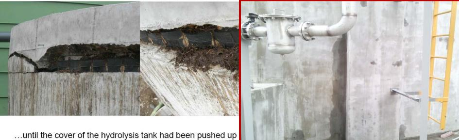
...until the cover of the hydrolysis tank had been pushed up fluid pressure and blasted from the tank.
