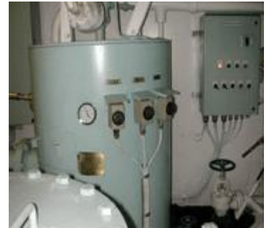
Hot Water Calorifier
