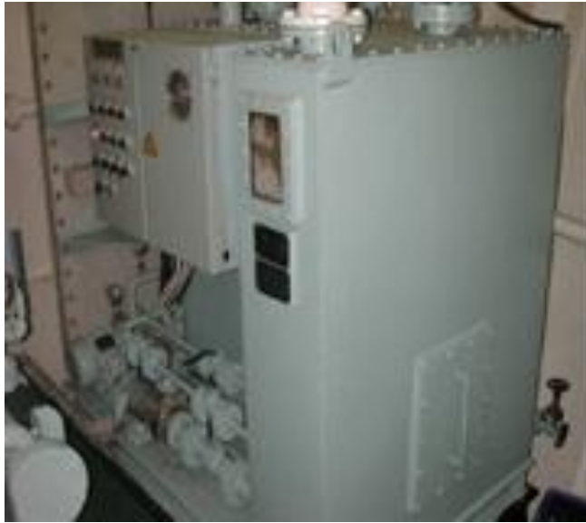
Swage Treatment Plant
