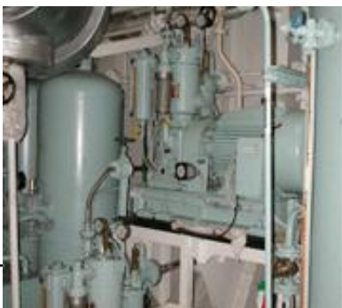
6. Main Air Compressor
