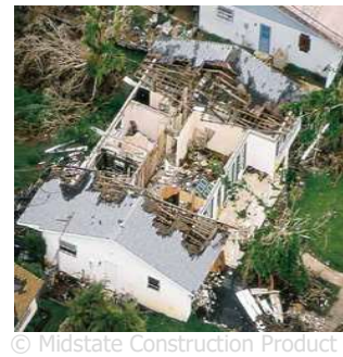
© Midstate Construction Product
