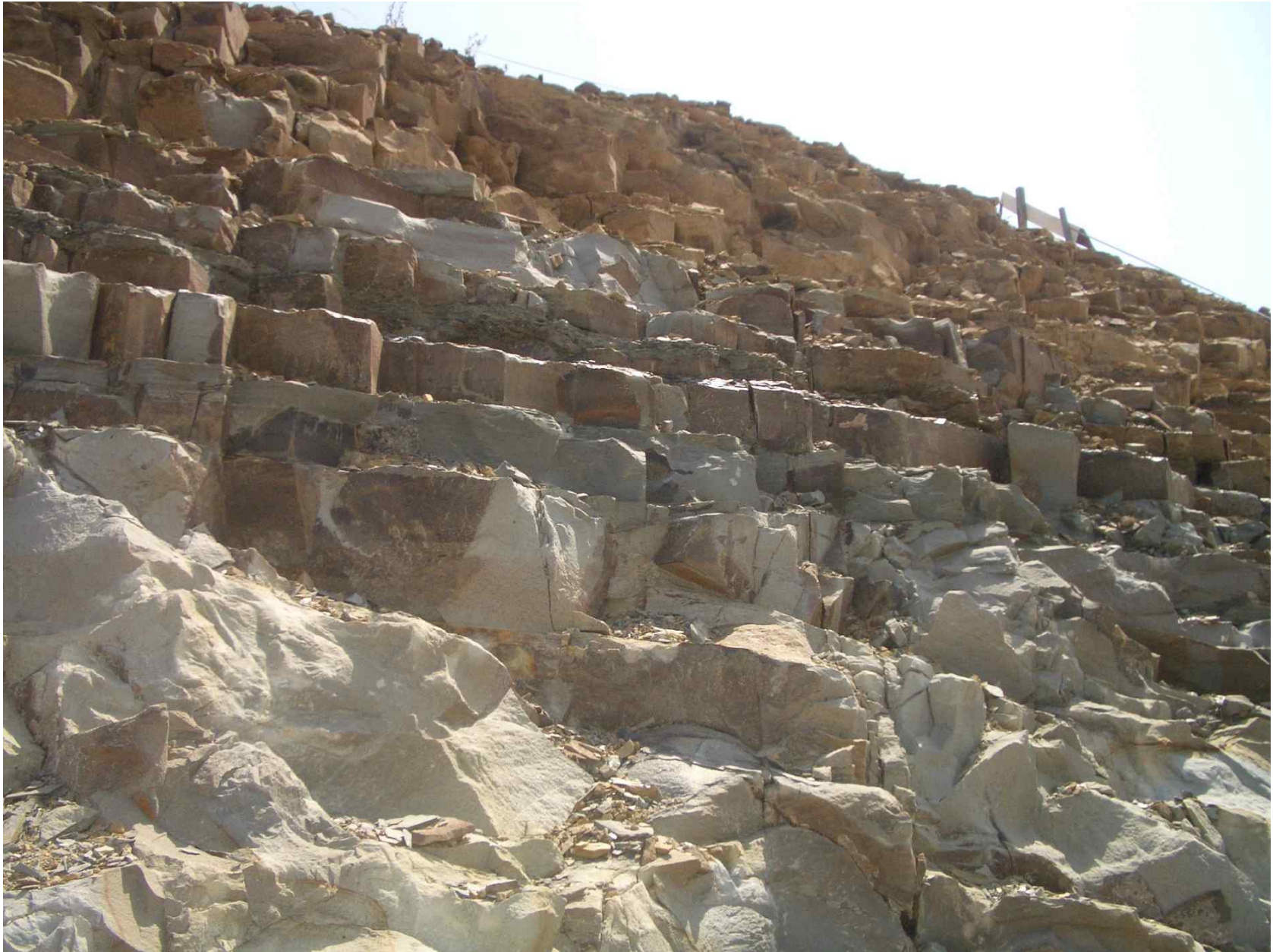
Analysis of rock mass discontinuities
