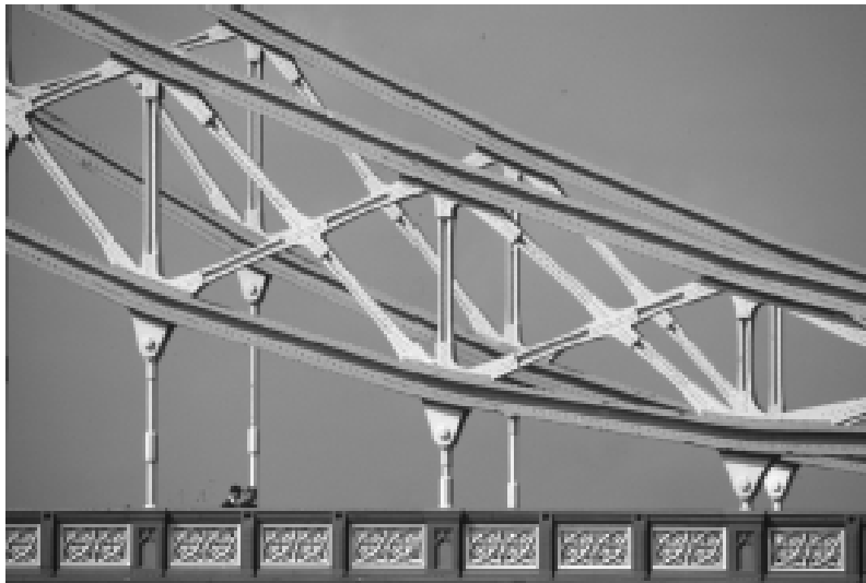
These steel tie rods, used to support a portion of a bridge, are subjected to tensile forces. Michael S. Yamashita/Corbis Images.
