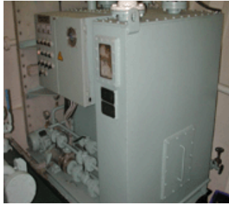
Sewage Treatment Plant
