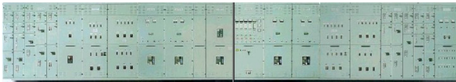
Example of switchboard
