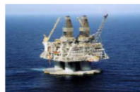
<Exploration and Production of the Natural Gas>
