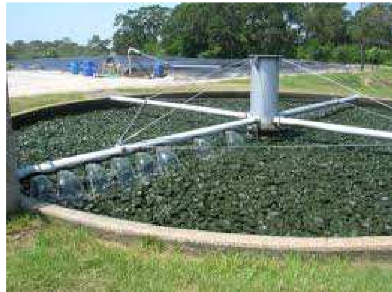
trickling filter
