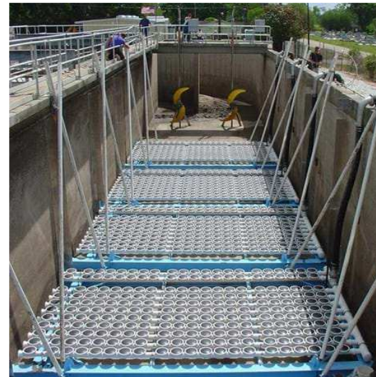
Installation of ceramic disk aeration devices to an aeration tank
