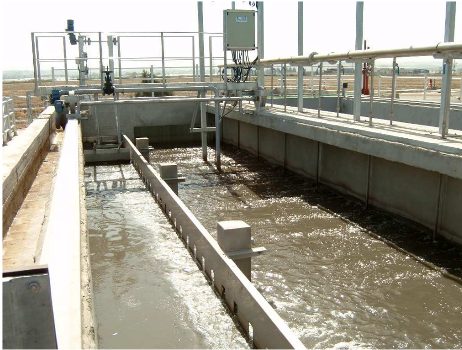
Rectangular horizontal flow grit chamber
