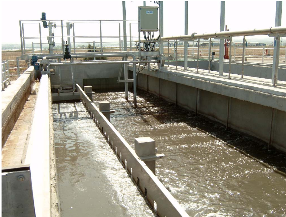
Rectangular horizontal flow grit chamber
