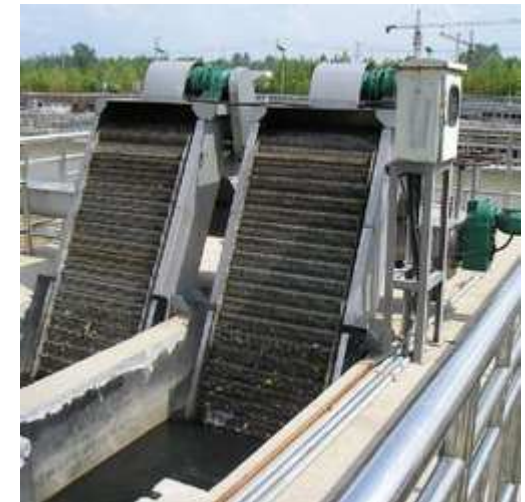
Mechanically-cleaned bar screen
