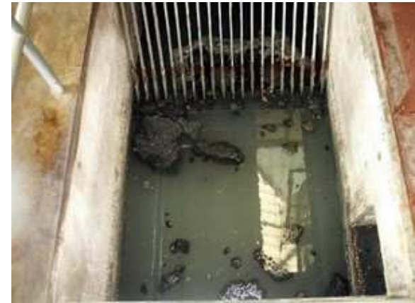
Manually-cleaned bar screen
