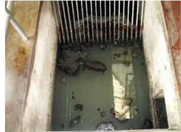
Manually-cleaned bar screen
