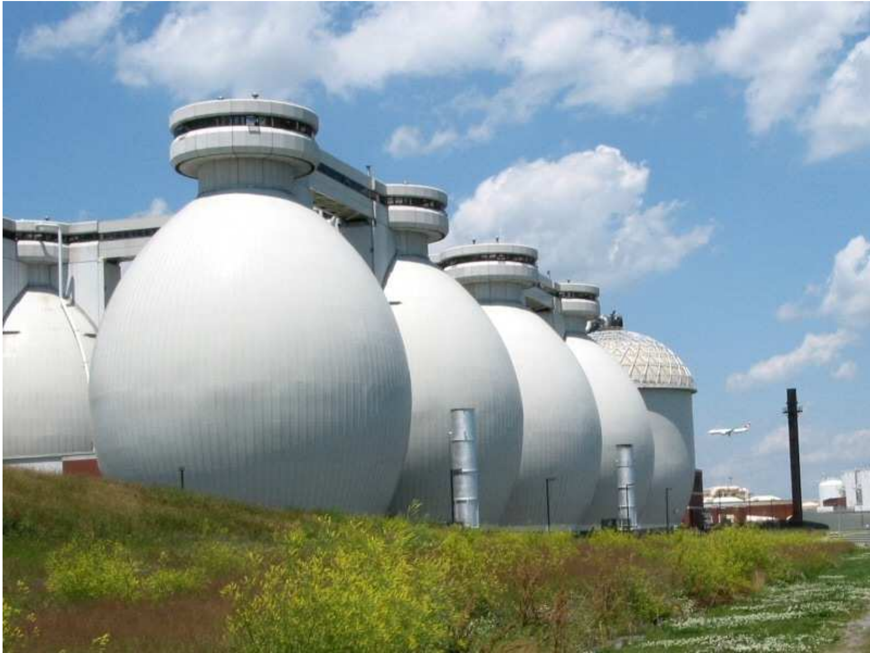
Dear Island wastewater treatment plant, MA, USA (sewage sludge)
