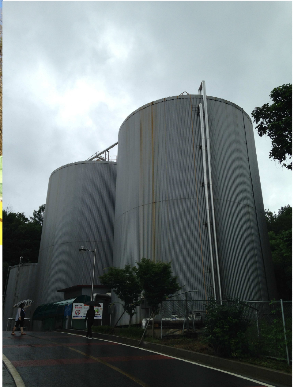
After construction (Feb 18)
