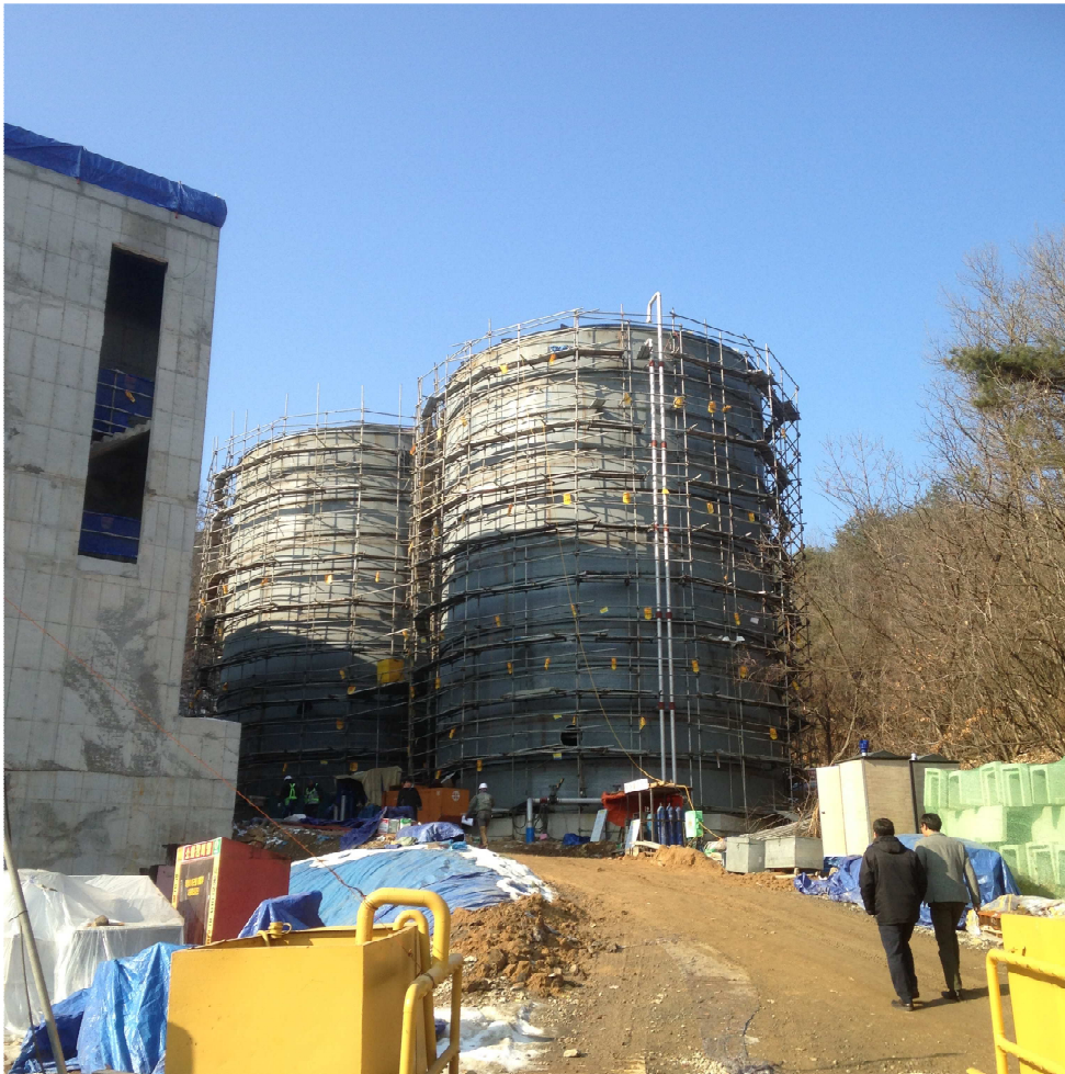
Before construction (Jan 15)
