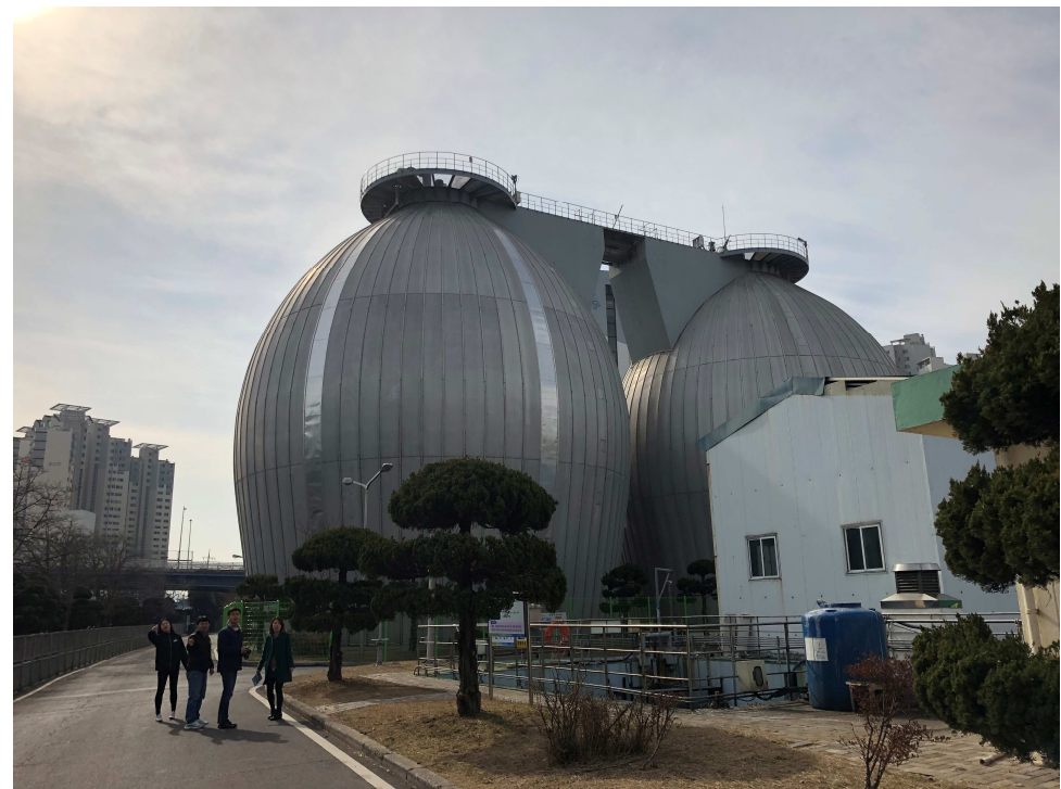
Biogas storage tank
