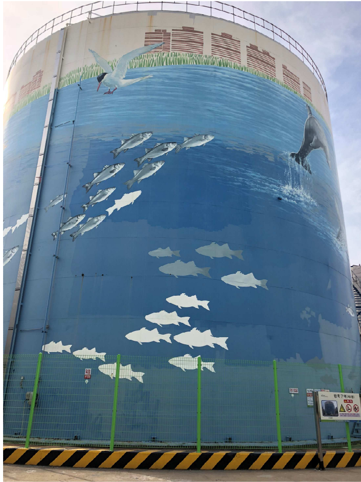
Anaerobic digestion tank
