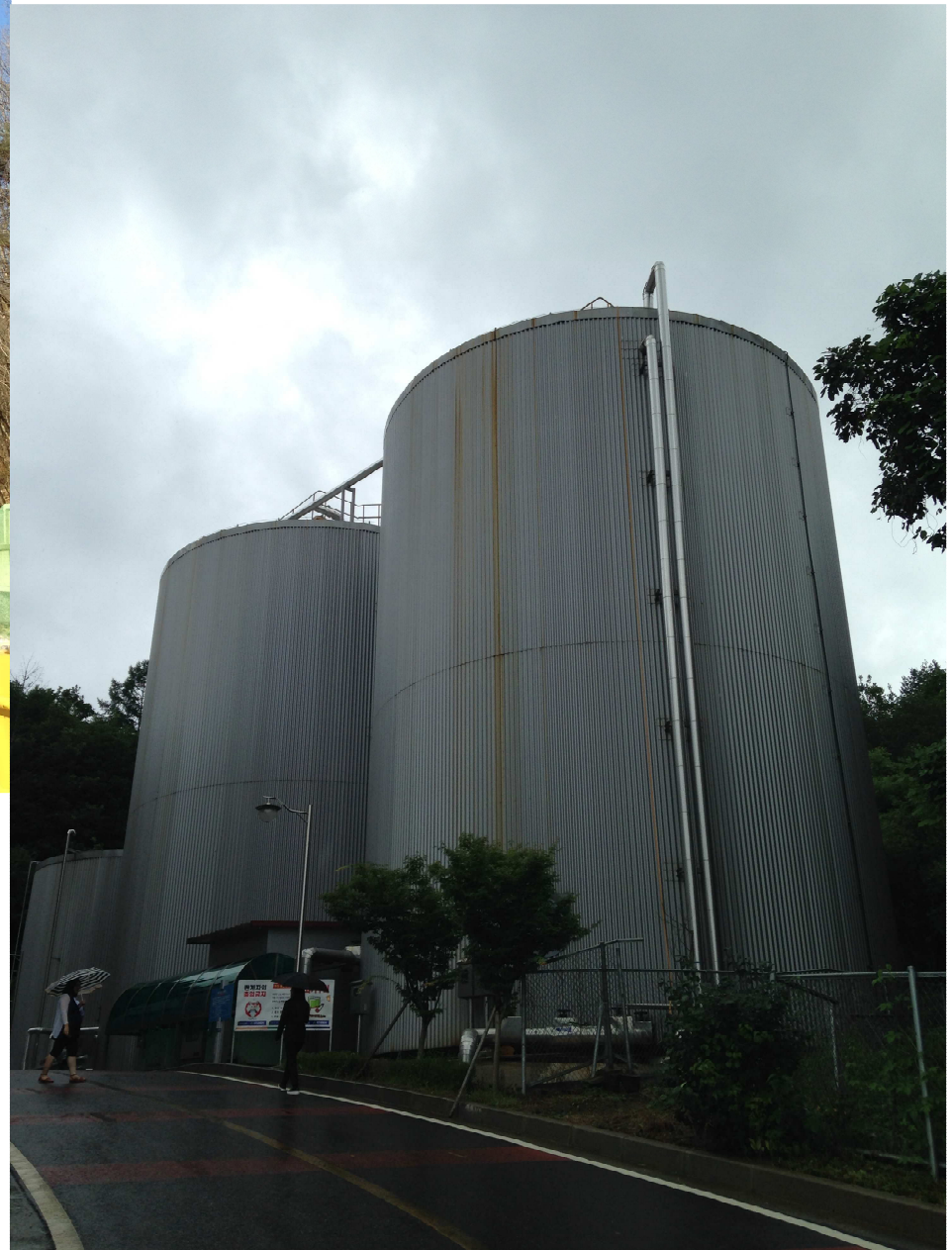
After construction (Feb 18)
