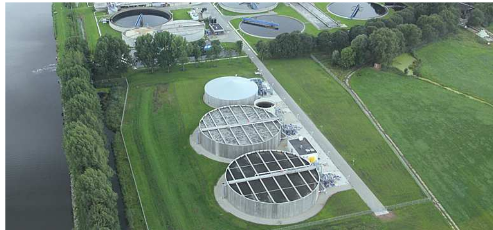
WWTP in Garmerwolde, the Netherlands (2010~)
