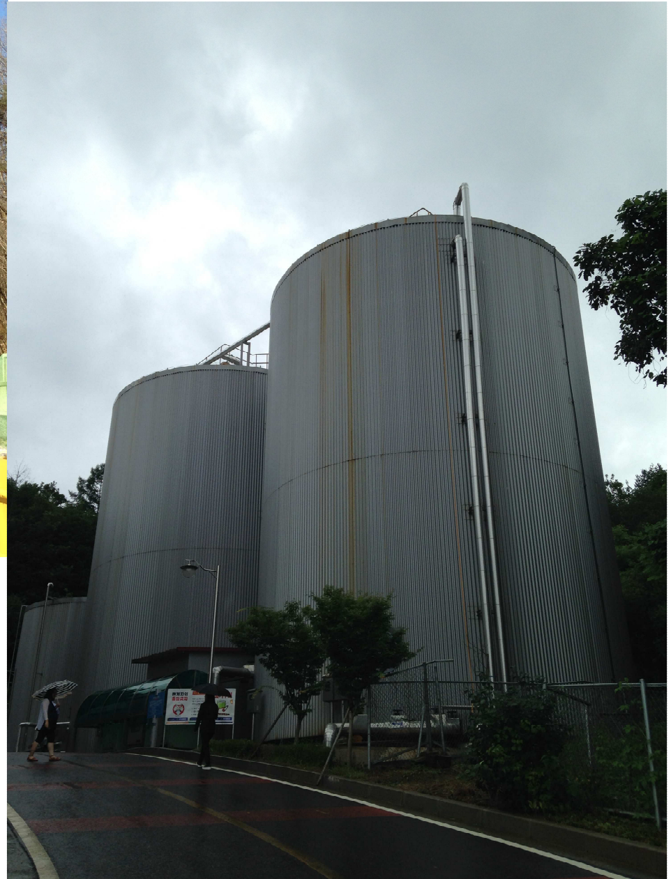
After construction (Feb 18)
