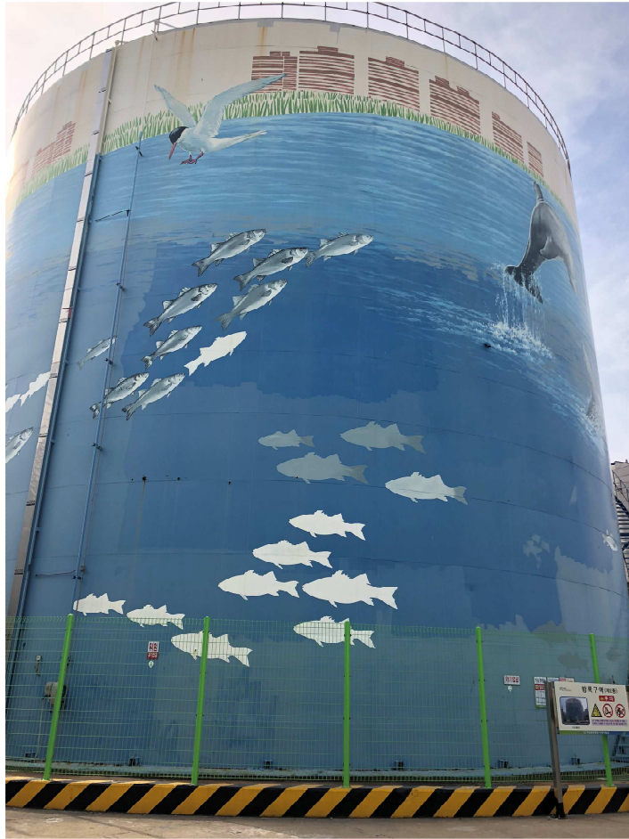
Anaerobic digestion tank
