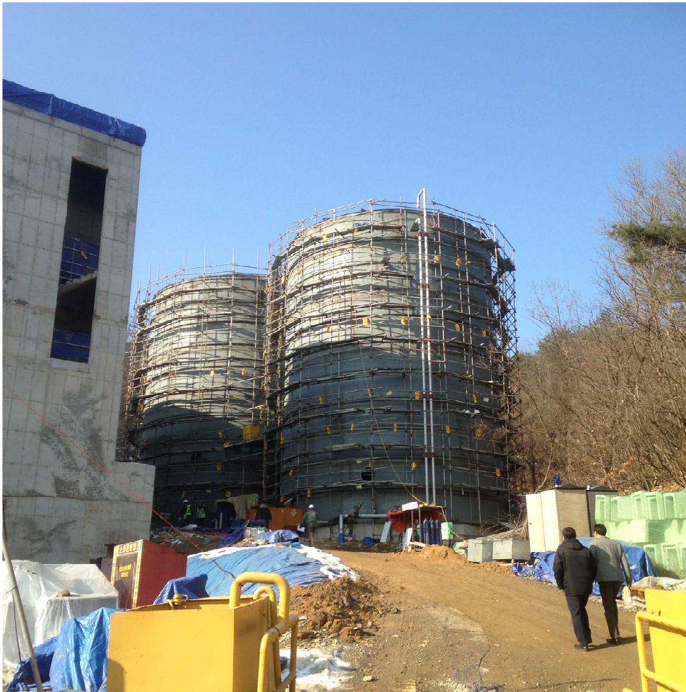
Before construction (Jan 15)
