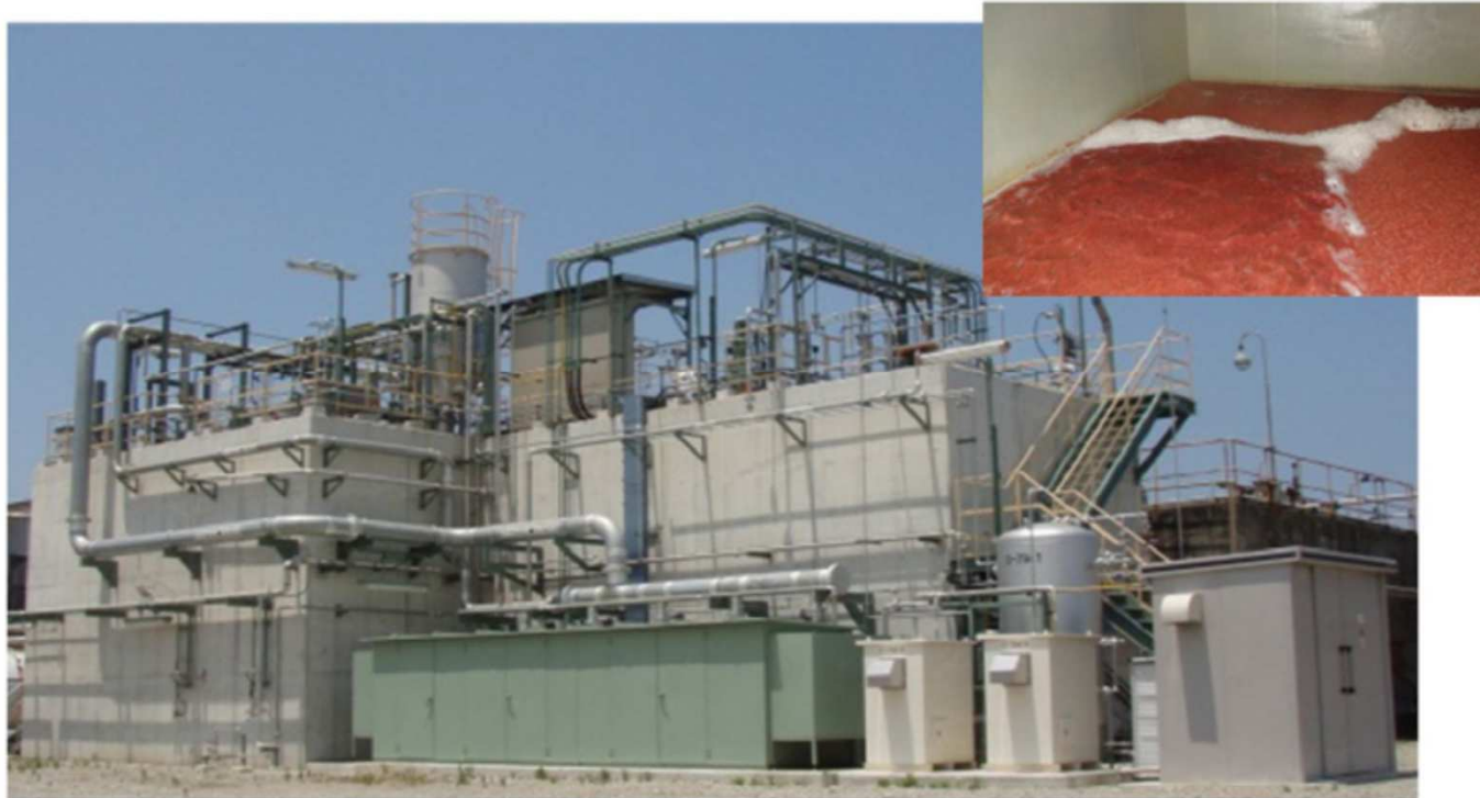
Fig. 1. (a) Schematic diagram and (b) photograph of full-scale anammox plant using gel carriers.
