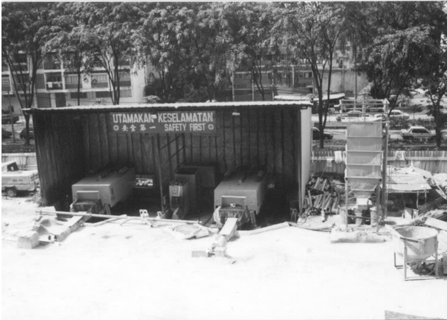
Stationary concrete pump
