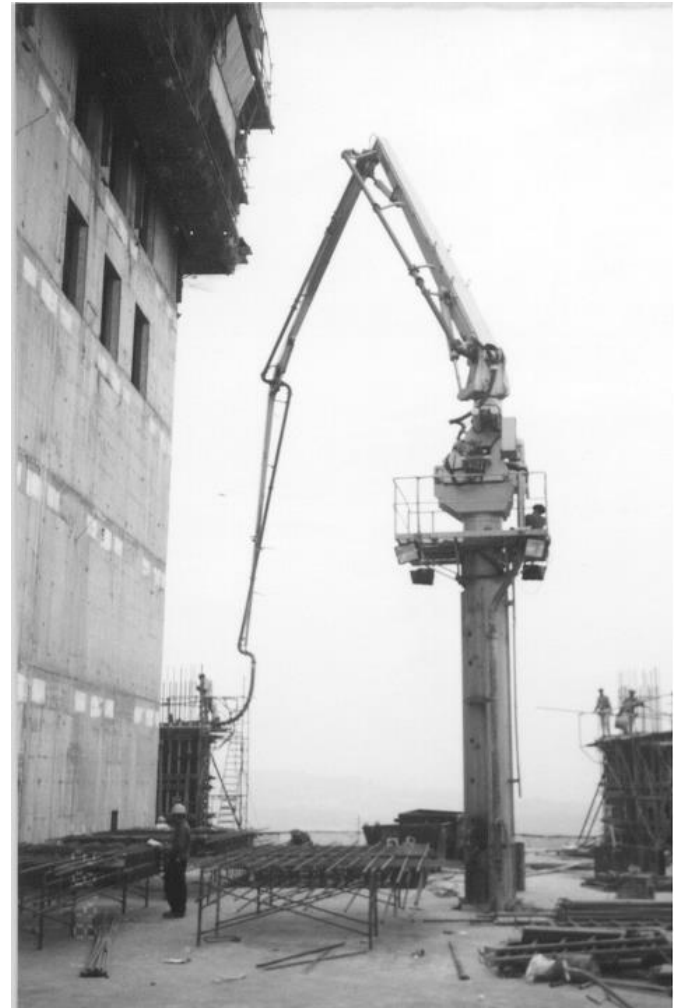
Concrete placing boom
