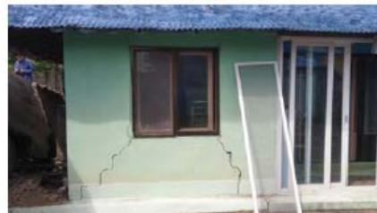
Typical corner cracking at opening
