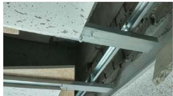
**Damage observed in a 3-story RC Building (Ulju, Ulsan)\_ ceiling and brick wall failure**
