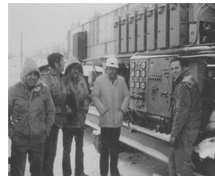
The first EGS power generation at Fenton Hill, USA(Feb, 1980, fluid temperature: 150°C, R-114 binary cycle, electricity capacity: 60 kWe, Armstead and Tester, 1987)
