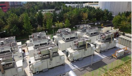
400 kW PAFC (PureCell) by Doosan Fuel Cell (formerly Clear Edge Power Inc)
