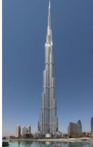
The Burj Khalifa, tallest structure in the world
