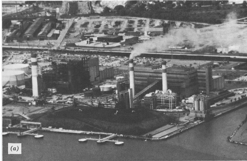
Coal burning power plant
