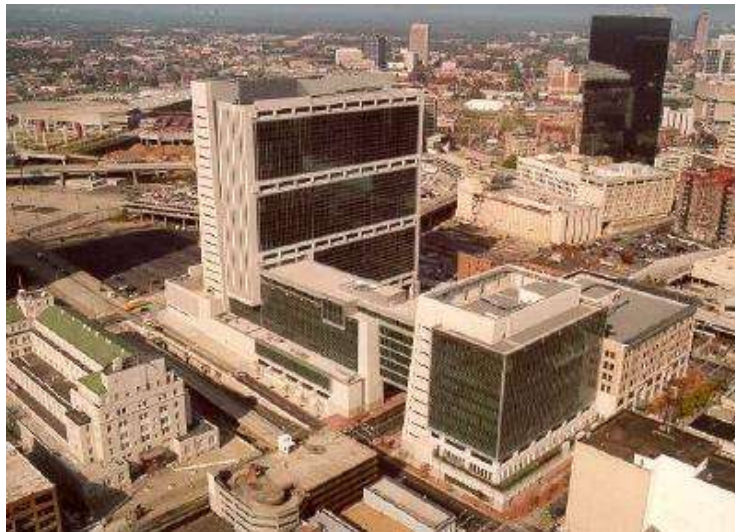
Atlanta Federal Center (total floor area = 145,000 m 2 )
