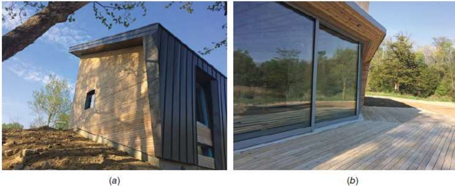
Fig. 1.10 (a) Construction phase photo of the west wall of the Iowa Nest. Design intent becomes reality during this phase, showing the shading of a deciduous tree on the west window on a summer day and (b) the shading of the high-performance, triple-pane sliding doors on the south-facing façade. (Photo © Carl Sterner; used with permission.)
