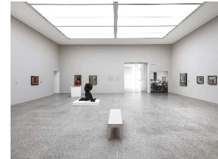
Example of luminous ceiling
