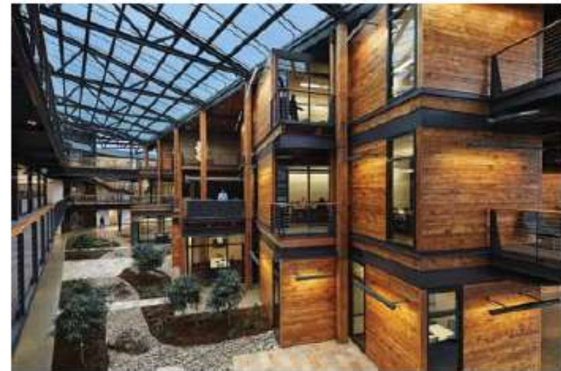
Fig. 11.10 Direct-gain atrium in the Federal Center South Building, Seattle, WA. (Image courtesy of ZGF Architects.)
