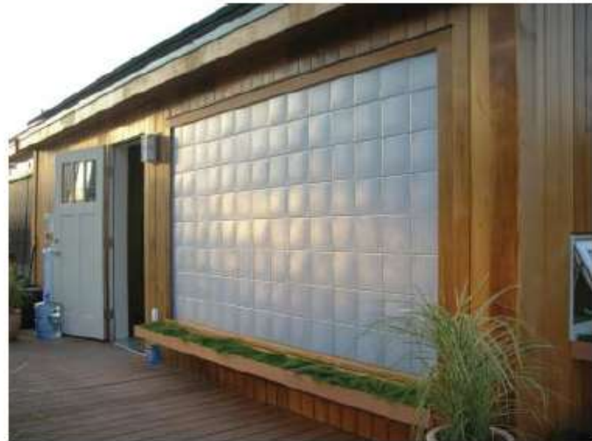
Fig. 1.23 Manage storage. The 2007 MIT Solar Decathlon house features a Trombe wall made of translucent tiles to capture and store heat. (© Alison Kwok; all rights reserved.)
