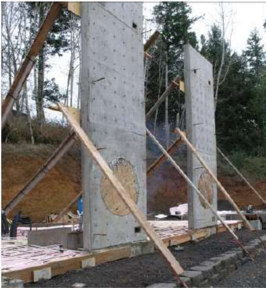
Fig. 11.18 A Trombe wall design for the Burger Residence in Lakeside, Oregon, completed in 2008, uses circular openings to preserve lake views. (Photos courtesy of D. Holmes Chamberlin Jr., Architect LLC.)
