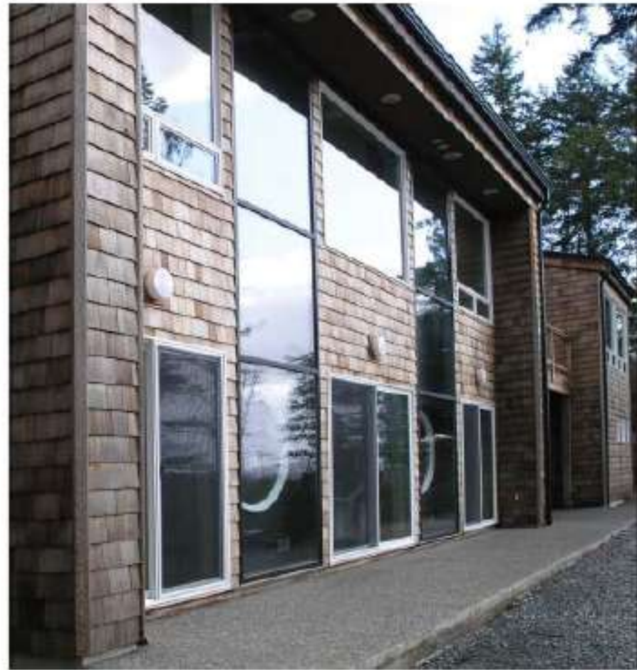
Fig. 11.18 A Trombe wall design for the Burger Residence in Lakeside, Oregon, completed in 2008, uses circular openings to preserve lake views. (Photos courtesy of D. Holmes Chamberlin Jr., Architect LLC.)
