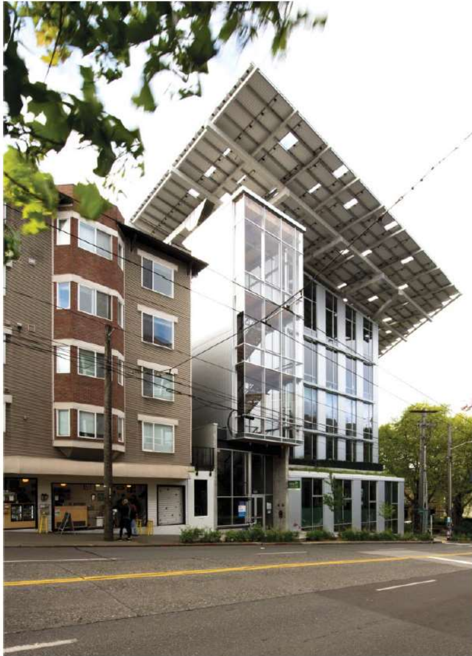
Fig. 2.10 Street façade view of the Bullitt Center, showing stairway, adjacent park, and cantilevering photovoltaic array. (© Miller Hull Partnership; used with permission.)
