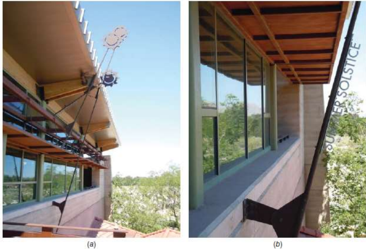
Fig. 3.40 Educational solar angles displayed (a) for a roof overhang at Springs Preserve, Las Vegas, Nevada. (b) Detail displaying the shade provided during the summer solstice. (© Alison Kwok; all rights reserved.)
