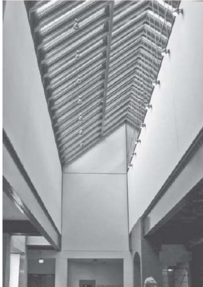
Fig. 10.18 Clerestory skylights with louvers at the U.S. Holocaust Memorial Museum in Washington, DC (Pei, Cobb, Freed & Partners). (© Alison Kwok; all rights reserved.)
