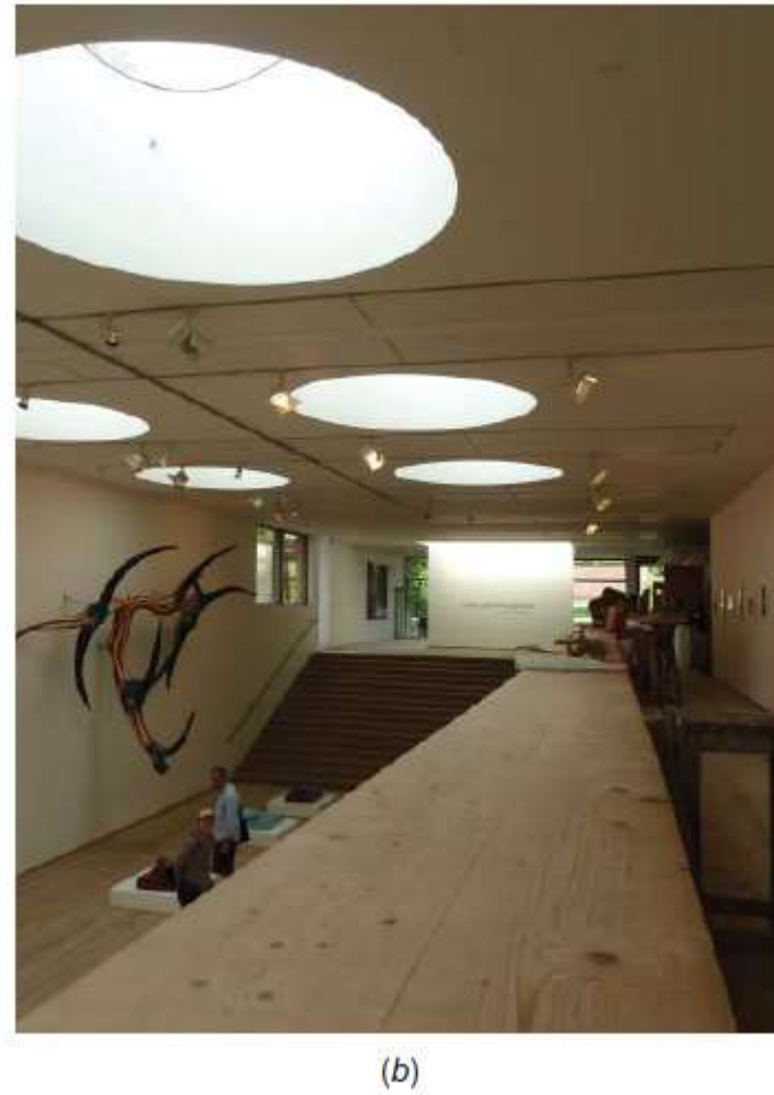
Fig. 10.15 (a) Splayed surfaces of a skylight provide areas for diffusely reflected light. (b) Conical skylights at Millesgården Museum and Sculpture Garden, Lidingö, Sweden (Everet Milles). (Drawing by Erik Winter; photo © Karen Tse; used with permission.)
