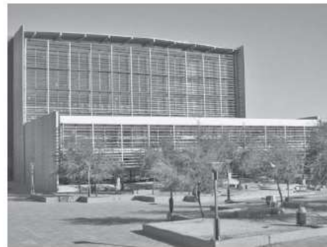
Fig. 10.14 Fixed horizontal louvers on the south façade at the Phoenix Public Library, Phoenix, Arizona. (© Walter Grondzik; all rights reserved.)
