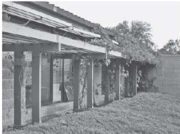
Fig. 9.1 The envelope is more than a surface. This south-facing office façade in Oregon forms a microclimate zone that buffers the transition between indoor and outdoor conditions. Groundcover plants at eye level for seated occupants and deciduous vines overhead give a seasonally changing view to the outdoors through a façade that also admits winter sun, year-round daylight, and summer breeze. (Photo by Amanda Clegg.)
